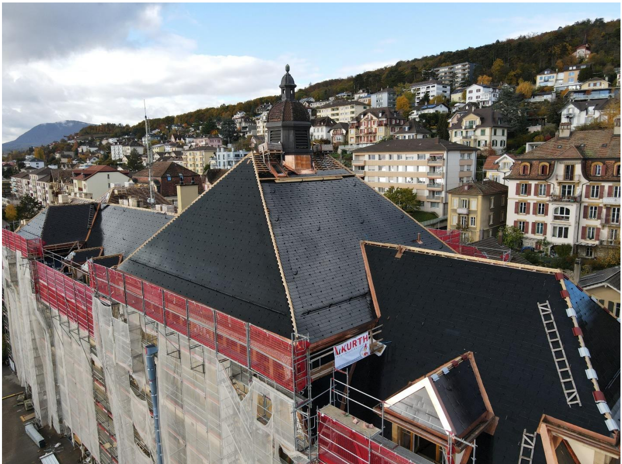
The Collège des Parcs in Neuchâtel, slated for completion in 2025, now features a dynamic solar-tiled roof, a collaborative innovation by Freesuns and CSEM.
